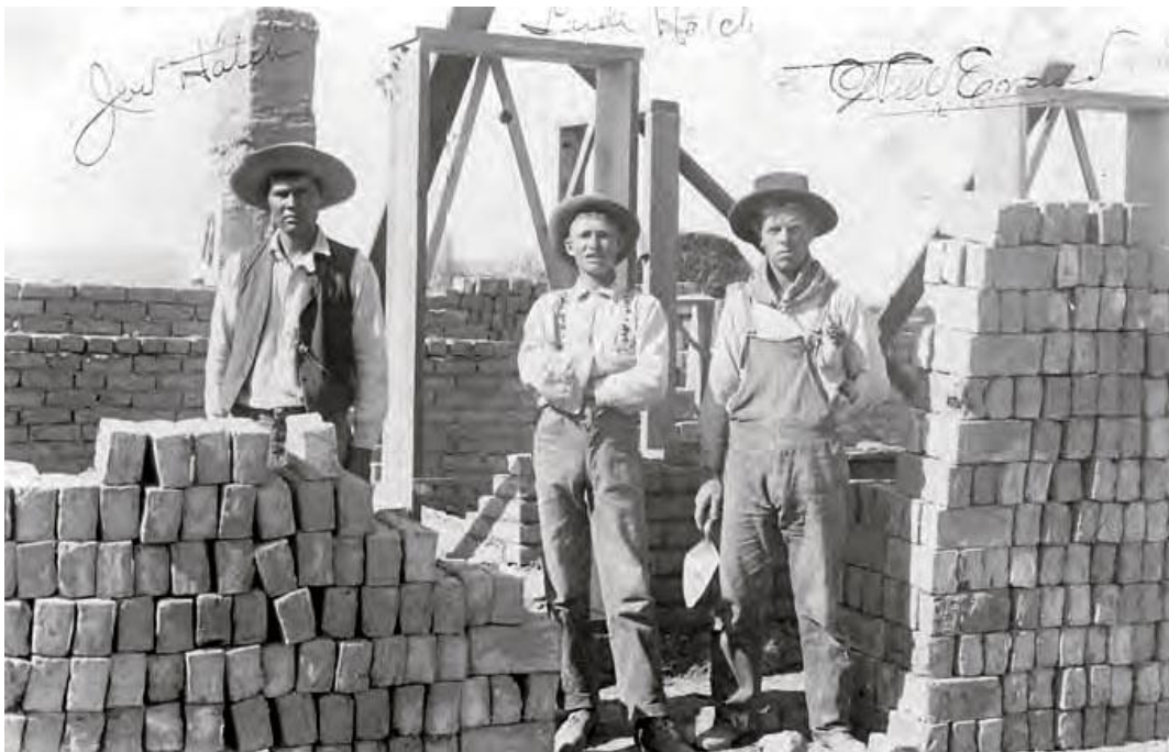
Joe Hatch, Sr. , Lude Kirk Hatch, & Will Evans building James 'Grandpa' Pipkin, Jr.'s house, June 1897, Fruitland, NM; shortly before Evans's initial trading experience at Sanostee. li
