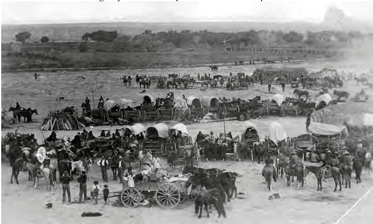
Ceremonial gathering in Shiprock, 1910. In the background to the right is a ceremonial hogan. Front left near the wagon tongue; a photographer has a large wooden camera on a tripod, focused on two men and an individual mounted on a horse. Shiprock Trading Post was a short distance to the left of this scene. lx
